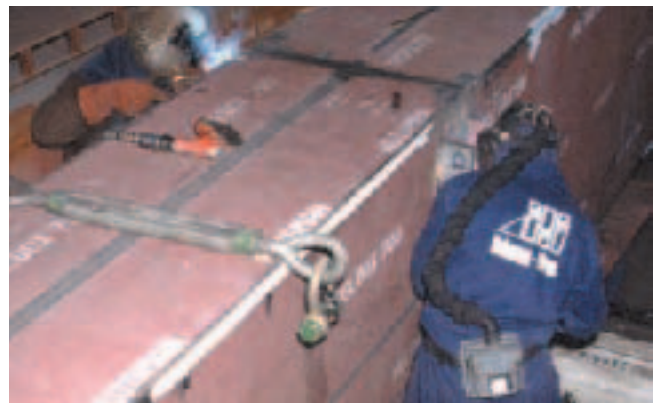
Figure 2. Vertically-up welding of a crane beam in Weldox 700.
