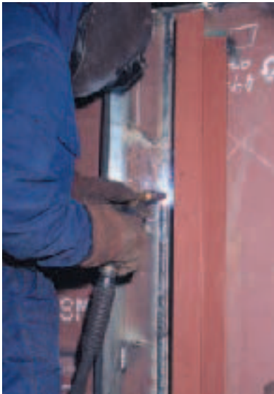
Figure 1. Vertically-up welding of a crane beam in Weldox 700.
