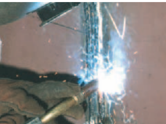
Figure 4. Vertically-up welding of a pedestal part.
