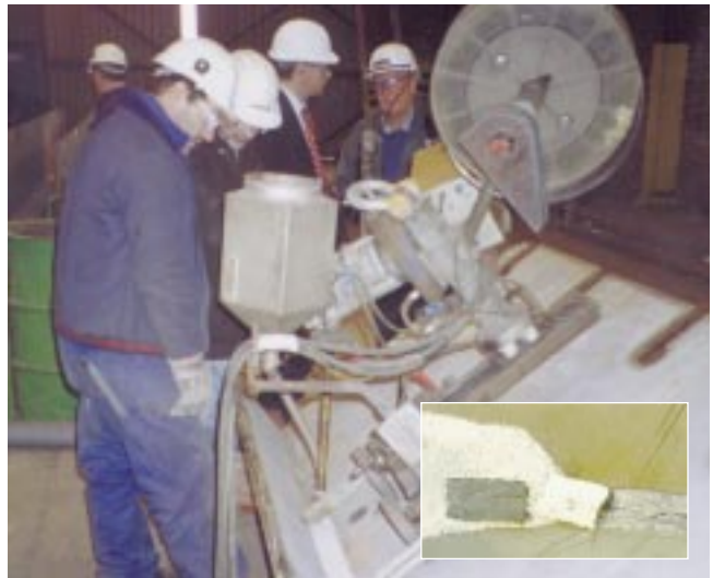
Figure 6: Fabrication of beams at KOG Methil.
